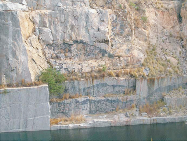
Figure 18. Leeukop quarry, 2 km north of the town of Paris, is one of the many dimension stone quarries that were operated in the 1980s and 1990s in the Vredefort Dome area. This quarry displays massive pseudotachylitic breccia and provides a glimpse of the geologic setting of mid-crustal granite-gneiss.
